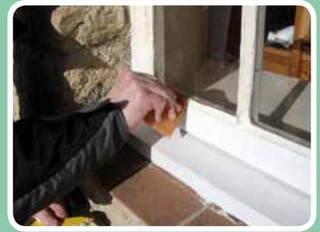
Replace failed linseed oil putty with DRY SEAL™ MP elastic glazing sealant
