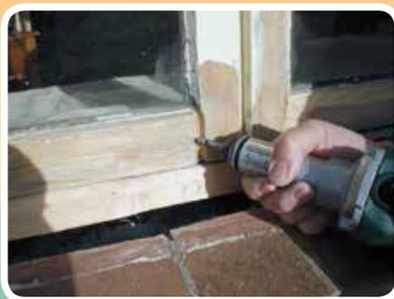
Seal construction joints, splits and shakes with DRY FLEX® resin
